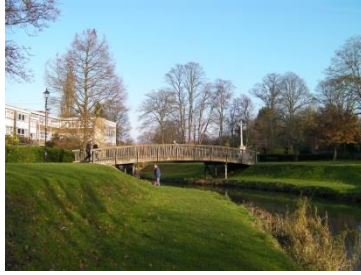
Bridge over a river
