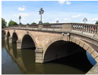
Traffic bridge over river
