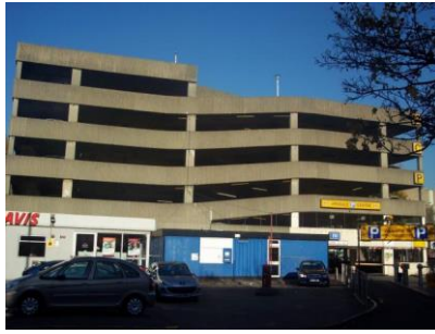
Multi-story car park
